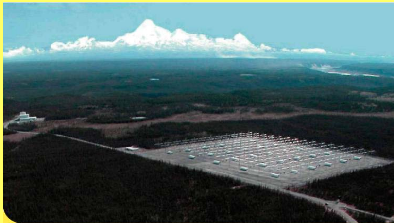
Fig. 25: HAARP location and construction.
